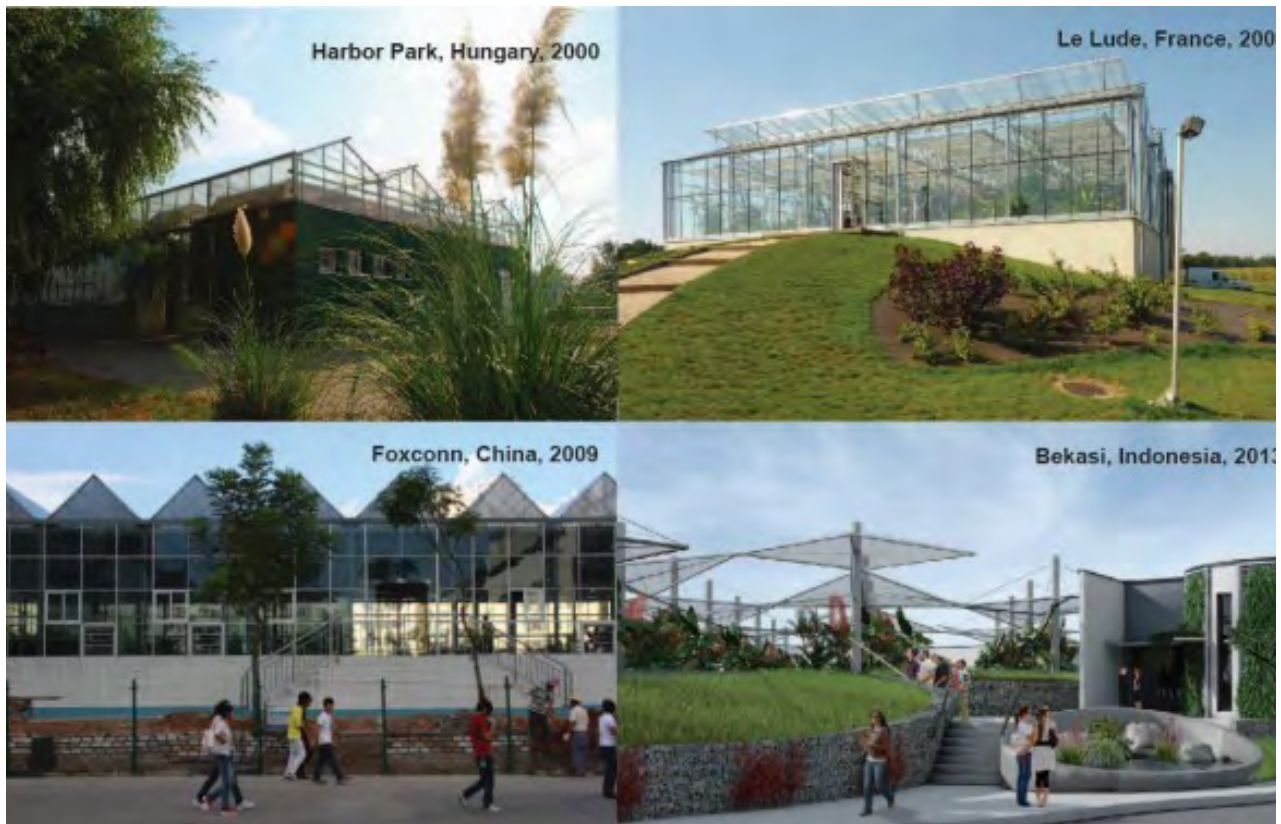
Organica Water's wastewater treatment plants in different cities (Source: www.organicaewater.com )
