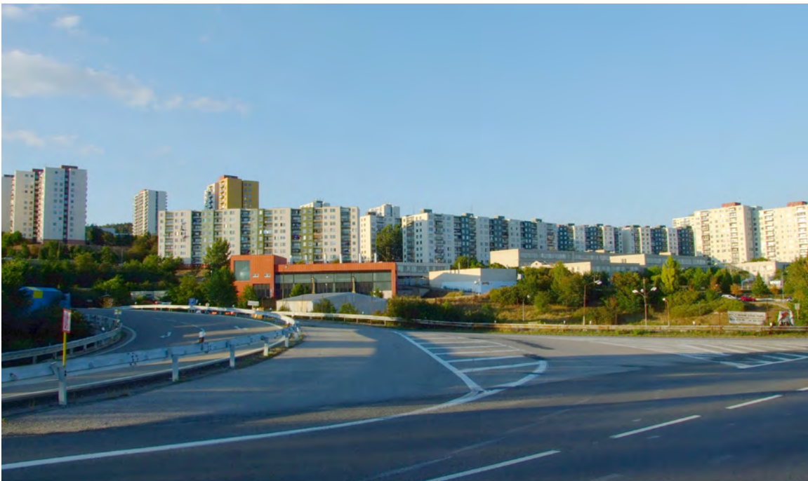
Prefab concrete apartment buildings in Nový Lískovec, Czech Republic, after renovation. (Source: Open license)
