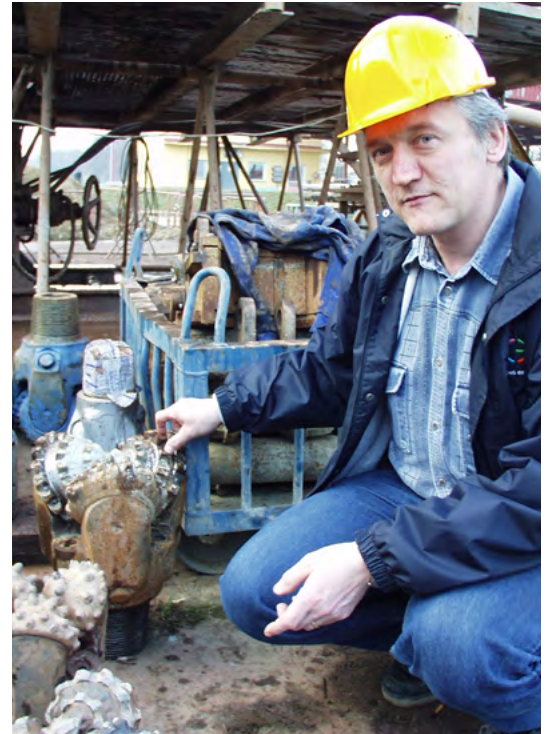
Drilling site of the geothermal energy project. The City of Litoměřice, Czech Republic (Source: The City of Litoměřice)
