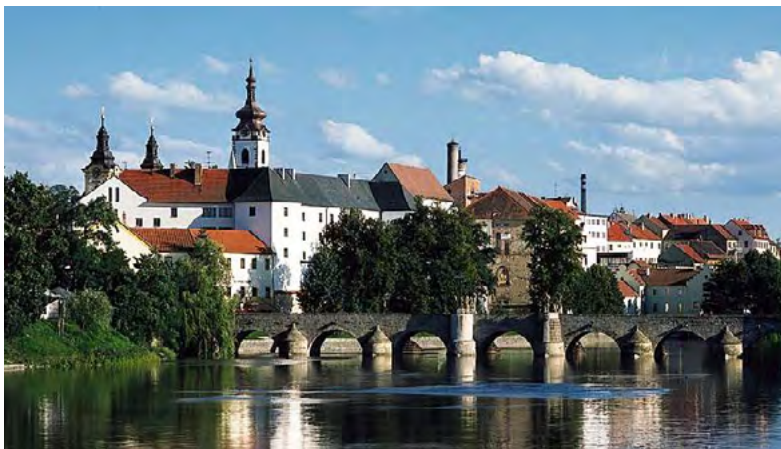
The oldest Czech bridge (from the 13th century) is located in the first Czech smart city. (Source: Open license.)
